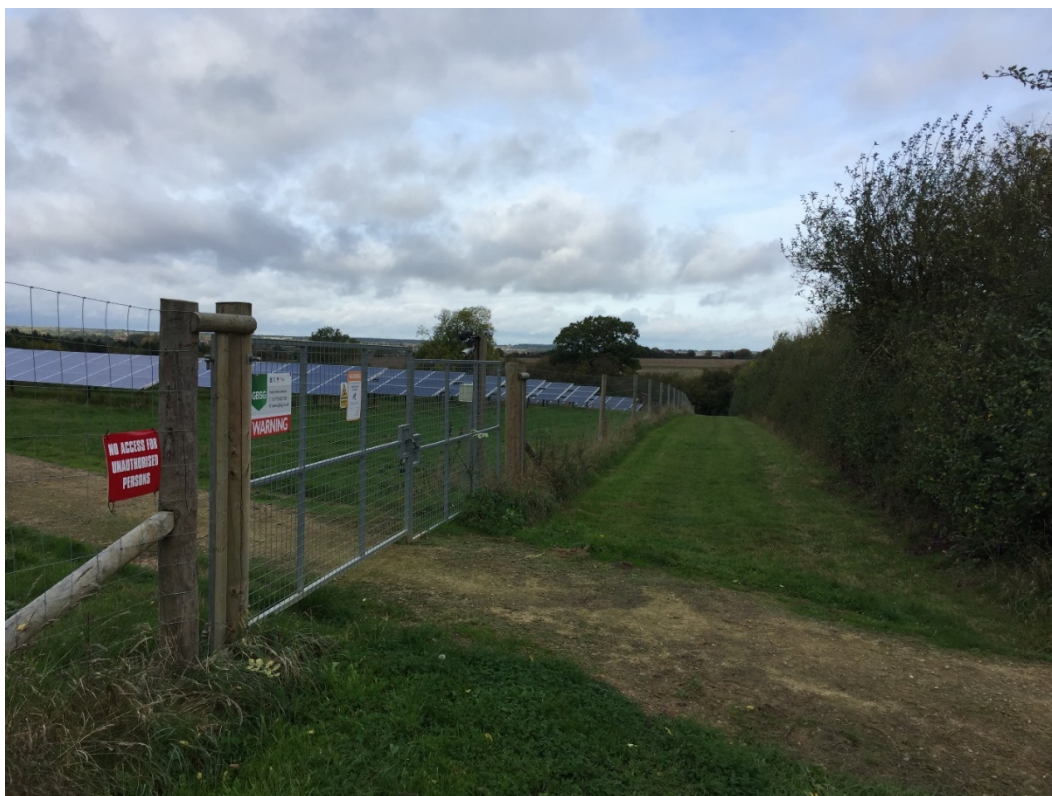
Plate 6 – Example image of a security fence, access gate, CCTV camera, internal access track.
