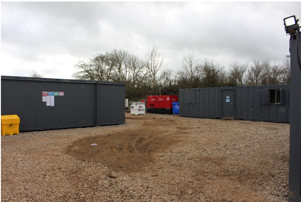
Plate 9: Establishment of the temporary construction compound(s)
