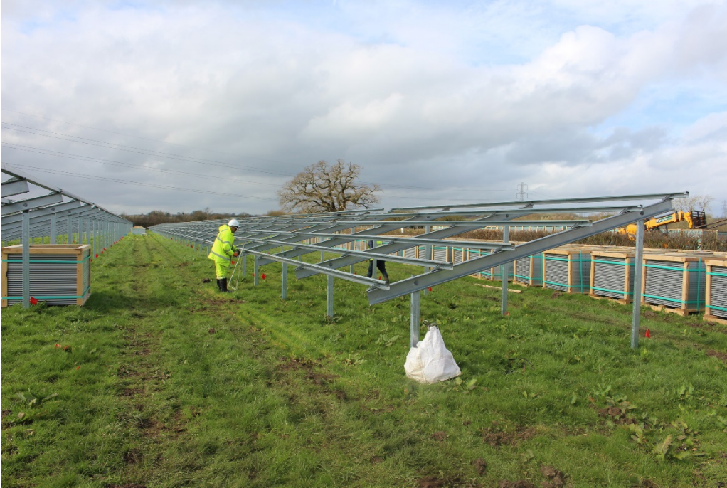
Plate 11d: Installation of Mounting Structures (4 of 4)
