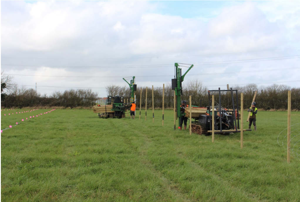
Plate 8: Establishment of Site fencing
