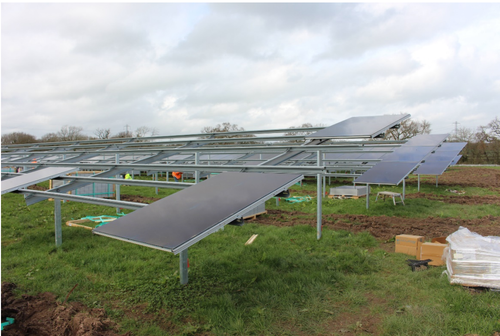
Plate 12: Mounting of PV Modules
